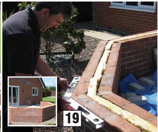
The dwarf walls are built to the height agreed and should include insulation in the cavity wall.
