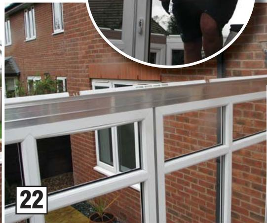
On completion of the frames the structural aluminium eaves beam is fitted to the head of the frames.
