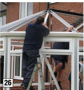
All the glazing bars are fixed from the eaves beam to the ridge.
