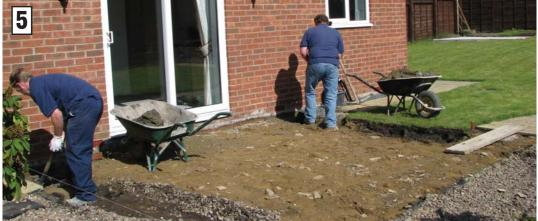
Construction work begins with the digging of the strip footings.
