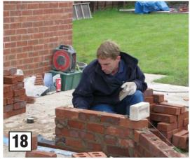
The remaining dwarf walls are built to match the existing brickwork or as requested by the homeowner.
