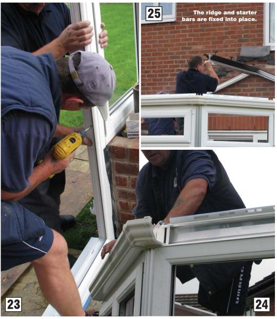
The doorframe is fitted to the side frames and dwarf walls.
