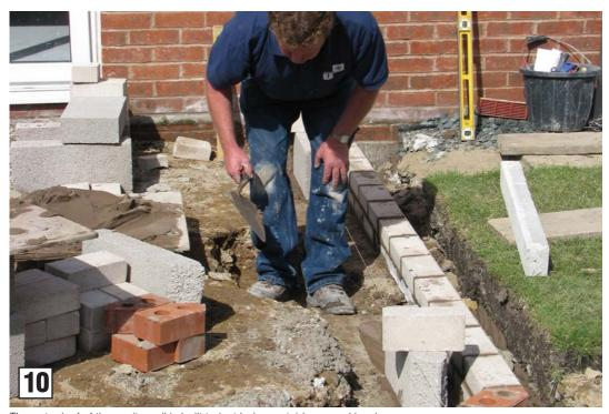
The outer leaf of the cavity wall is built to just below outside ground level.
