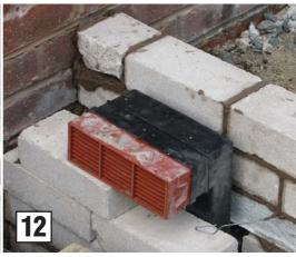
Any existing air bricks can be transferred through the base work.
