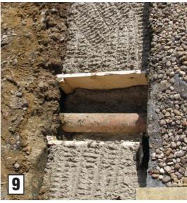
Any drainage pipes will be identified, protected and 'bridged' by concrete lintels.
