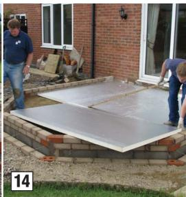
Floor insulation and a damp proof membrane are laid over the sand.
