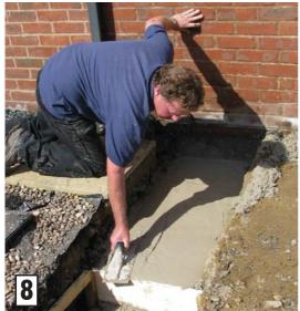
The concrete is floated to form a level surface area to build upon.
