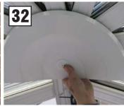
The PVC internal cladding are clipped onto the eaves beam and ridge to complete the internal trims.
