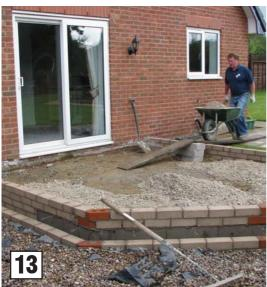
Hardcore is laid and compacted to a minimum 100mm deep. A blinding screen of sand is laid over the hardcore.
