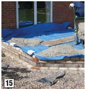
Concrete 100mm thick is laid to bring the slab up to the finished floor level.
