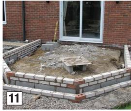
The inner leaf of the cavity wall is built to inner floor level.
