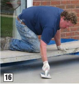
The concrete is floated to a smooth surface level.
