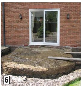
Footings are dug to a minimum depth of 450mm - this will vary depending on the ground conditions.
